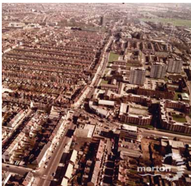
Aerial view Merton High Street - High Path Estate near completion in 1982
