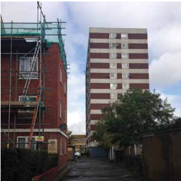
12 storey tower block on High Path Estate
