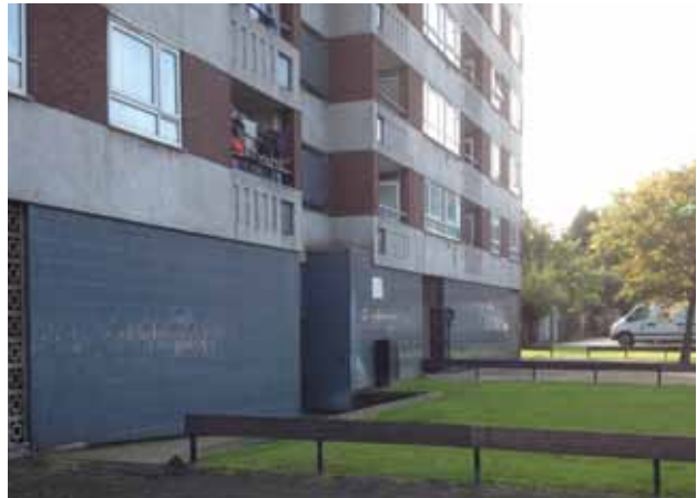
Unclear communal entrance with blank street frontage
