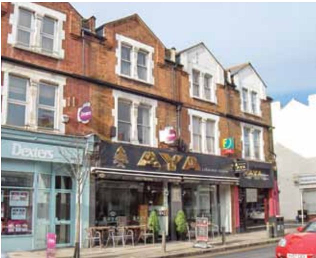
3 storey commercial buildings fronting Merton Road
